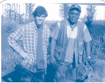
Joshua with a co-worker at a newly installed clean water outlet.
